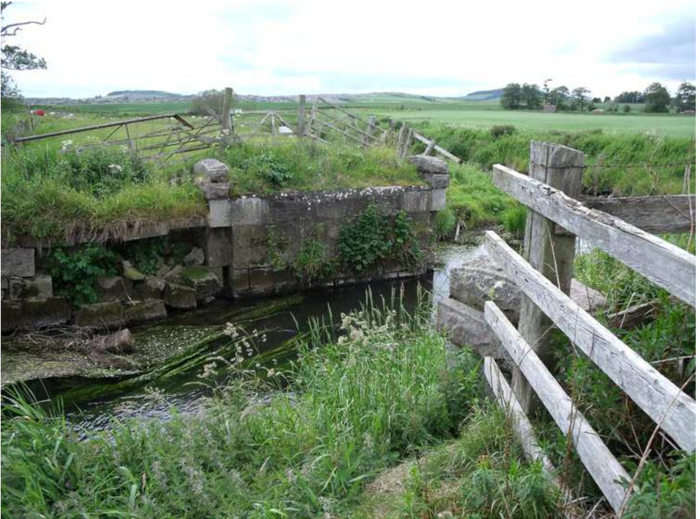
Flood damage to the existing bridge structure below Collyhill. This will need to be repaired. SEPA need to be informed as hard engineering is required. A rat or a water vole was spotted just to the left on the bank in this picture. A rat is no problem but a water vole presents conservation issues. OS Ref NJ 768 240
