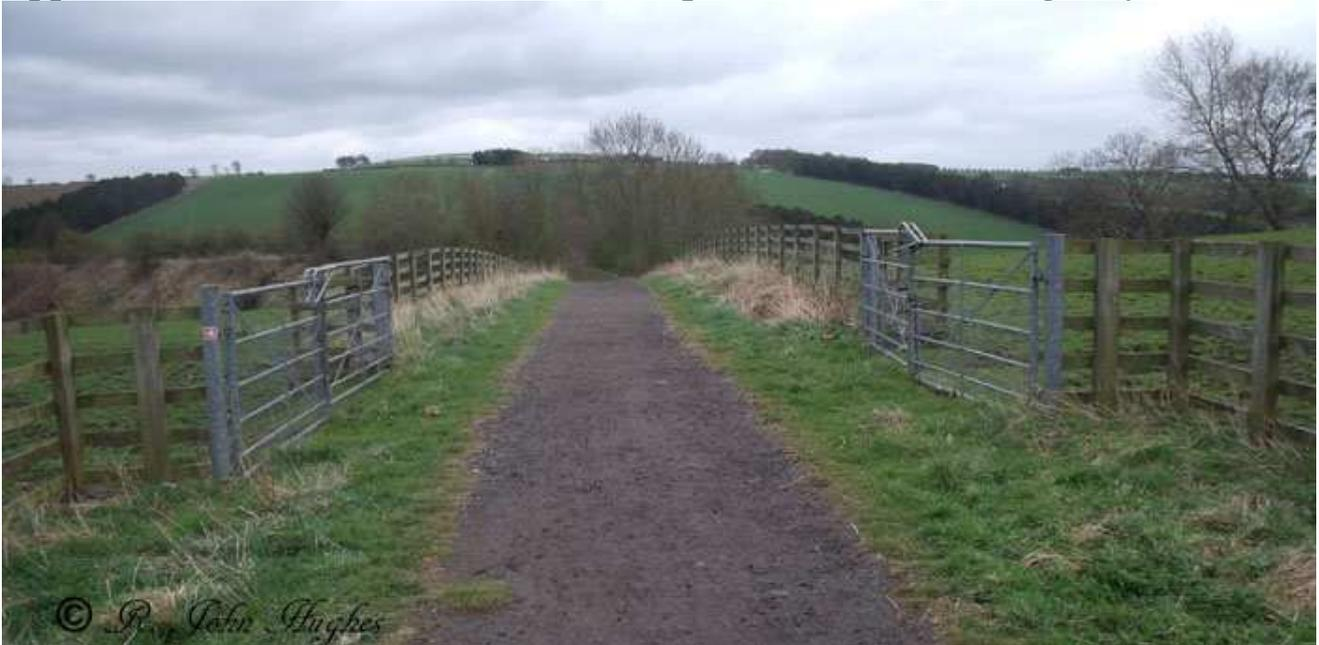
Above Sustrans route 14 near Lanchester, County Durham showing wooden and rylock sheep fencing (outside of track side). This would be the standard required for roadside tracks and tracks going through fields with stock like sheep and horses in. For Cattle a further barbed wire fence high on field side might be required.
