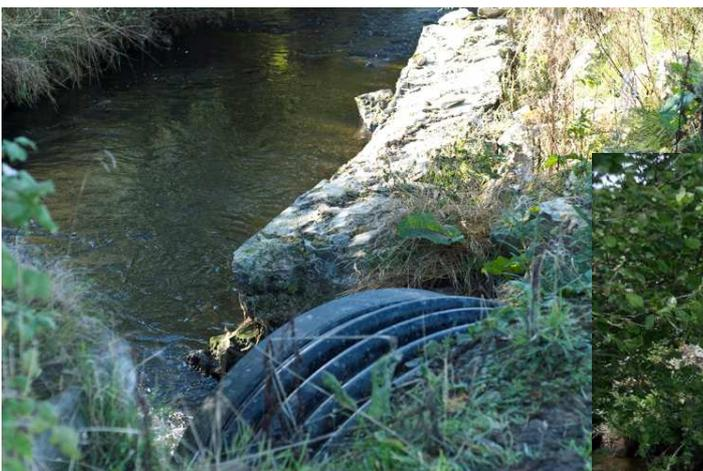
Damage on the west edge of Lochter caused by flood damage and poor engineering in the construction of a large bridge/culvert will require to be repaired.
